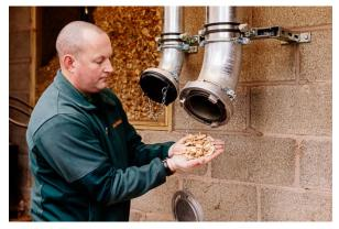
Woodchip is delivered straight from the delivery truck by air pipes connected via a lipped-end pneumatic air coupling to JACOB 150 mm diameter galvanised modular pipework, straight to the customer's woodchip store. The advantage is a saving on overall height as there is no overhead auger required, achieving a more even fill as the air system delivers woodchip evenly across the storage area.
