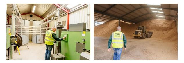
After processing as woodchip, the fuel is dried to reduce the moisture content to 20-30% depending on customer requirements. Edge Renewables currently supply around 30,000 tonnes of woodchip annually.
