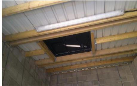
*The purpose built roof hatch with electric operation for loading wood chip with our specially designed delivery lorry.*
